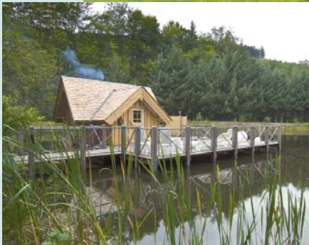
New Sauna on pillars in Swimming Lake
